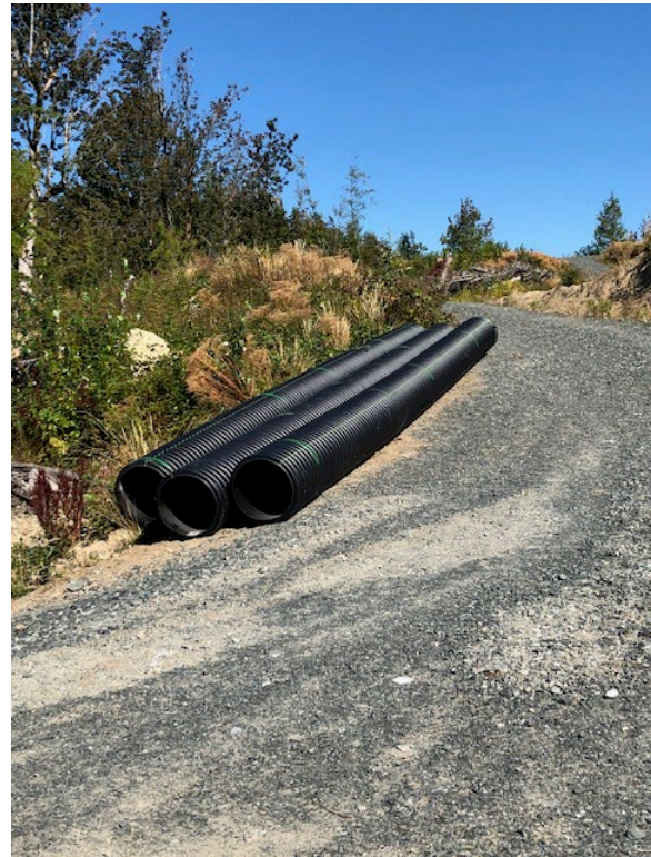
Figure 2: Road and culverts on Samish Heights (2020)
